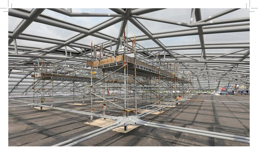
The scaffold frame was left exposed directly above the timber protection so the birdcage scaffold could be set out from the bridged support and extended to the full height.
