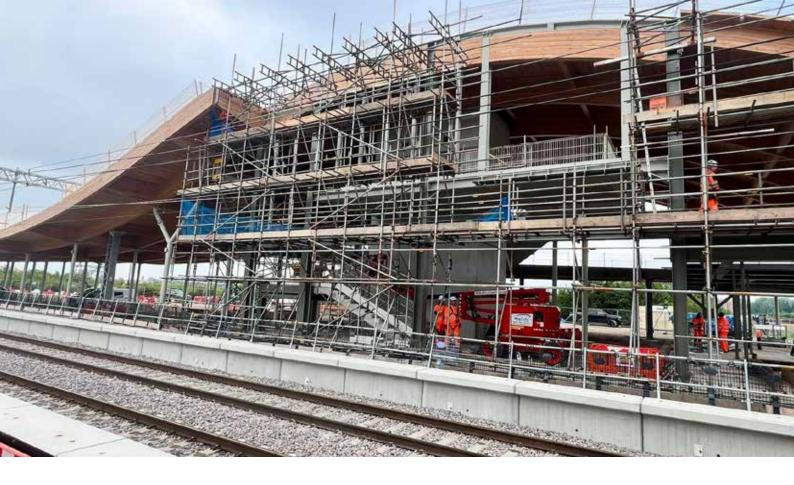
The purpose of the scaffold was to provide access for the installation of glazing panels that make up the building's façade.
